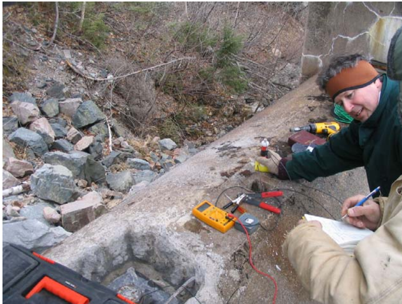
Figure 5: Half-Cell Potential Measurement in Progress
