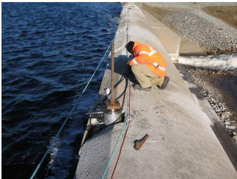
Figure 7: Installation of additional rock anchors at Log Falls Dam, 2006.
