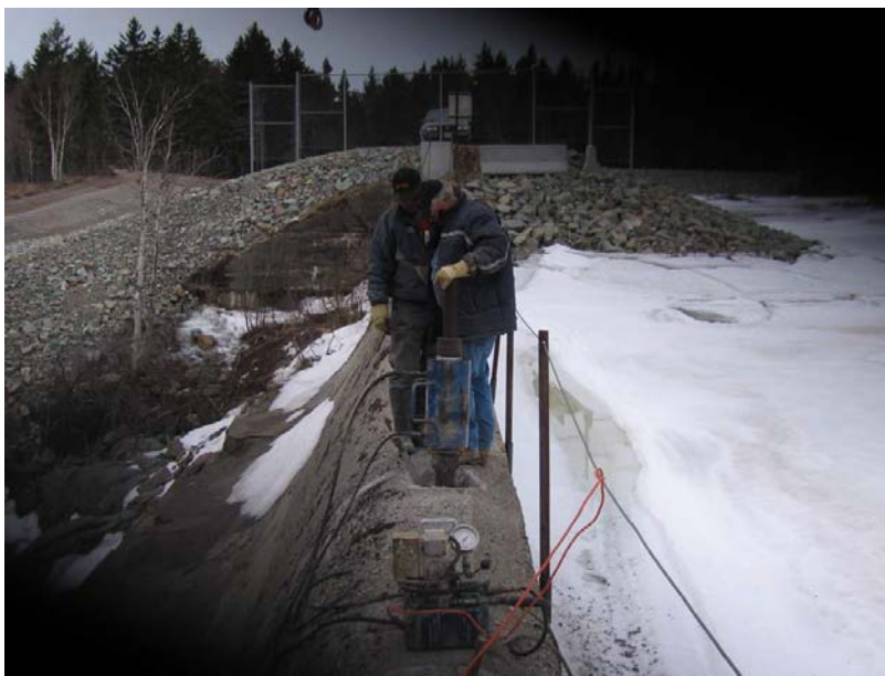
Figure 4: Lift-Off Test in Progress at Log Falls Dam
