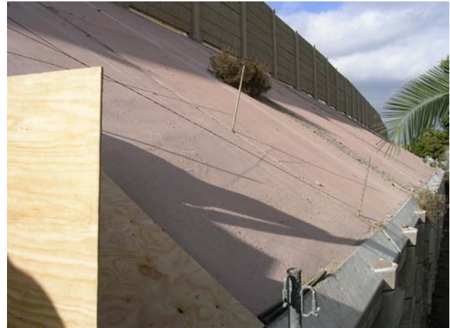
FIGURE 2(b). Wall #3 Supporting I-515 Embankment North of Flamingo Rd. On Ramp.
